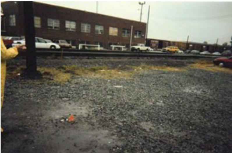
Photograph 3 After treatment the injection points were left in place but cut off at ground level.
