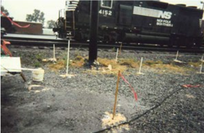
Photograph 2 Injection points within 4 feet of train tracks as trains pass by.
